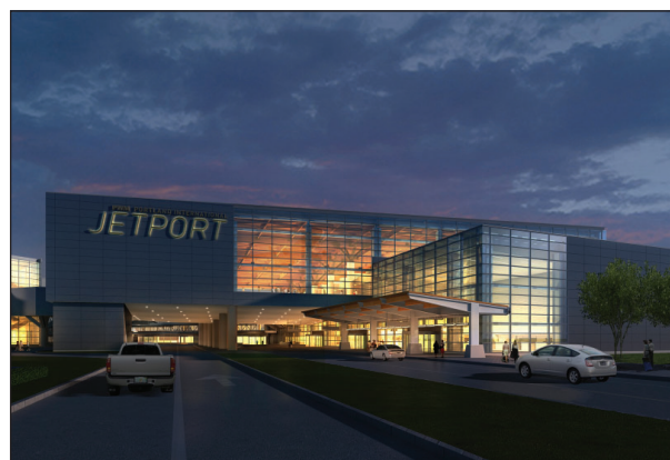
Airport Terminal Expansion - Portland, ME
