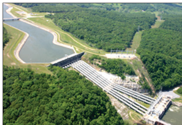
Grand River Dam
